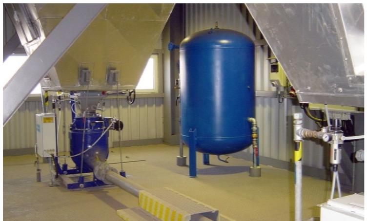
Primary vessel showing conveying air supply
